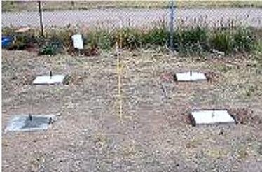
We mixed the 80 lb. bags of pre-mix one at a time in a wheelbarrow, using a garden hoe and a hose. We had to keep going until it was all done, so there would be no faults in the concrete, but eventually we poured the 4 footings, one for each anchor bolt. Each hole took 3 to 4 bags, so we have around 1100 lbs. of concrete in the ground. We kept the concrete covered for several days while it cured, wetting it occasionally. After it cured,
