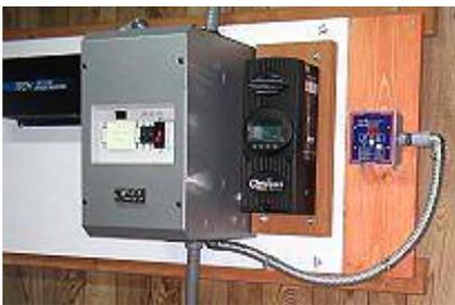
The equipment plate roughly mimics the layout of a pre-wired **Outback Power Center**, since we are using two **Outback** components. The **DC breaker panel** is in the center, with the **charge controller** directly to the right, and the **Exeltech Inverter** on the left. There is room for a larger inverter. We marked and drilled holes beforehand for “T-Nuts”. These grab the plywood on the back surface, so the equipment can be mounted to the front with machine screws. We mounted the
