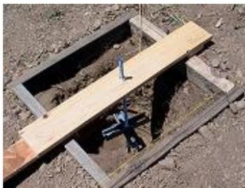
We built some 20-inch square forms out of old 2x4's to finish off the tops of the holes. Then we made an anchor bolt template out of
