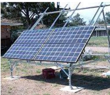
The top-layer rails on the tilt-frame run up and down, in two pairs. Side-to-side spacing is infinitely adjustable, since the rails are attached to lateral channels underneath with channel nuts. We spaced the top rails to match the mounting holes in the module
