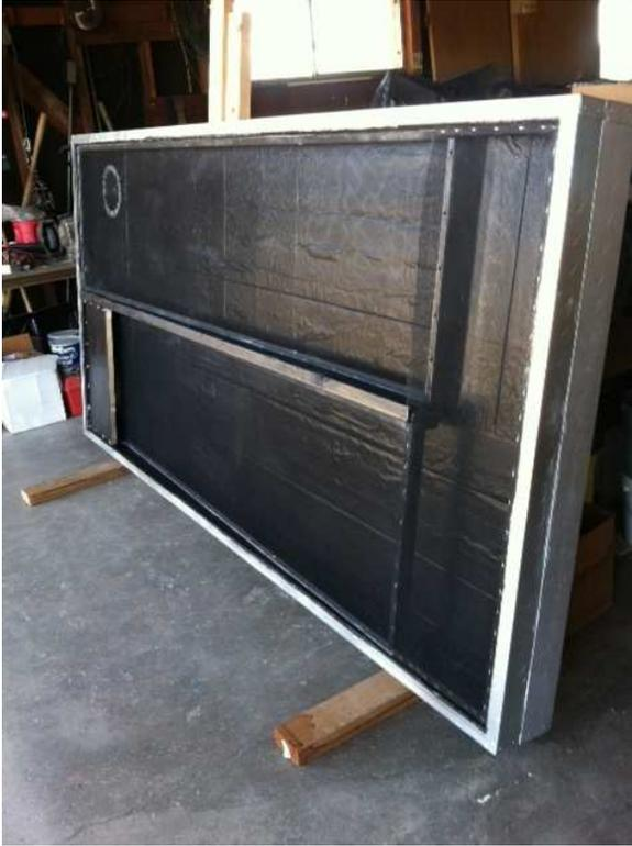
The 2x4 blocks fitted into the stud track were sort of a compromise; they created too many thermal bridging paths to the outside. Reconsidering, it may have been better to first insulate all around with 1 in. polyiso, and then fit an inner frame made from 1x4's for the screens.
