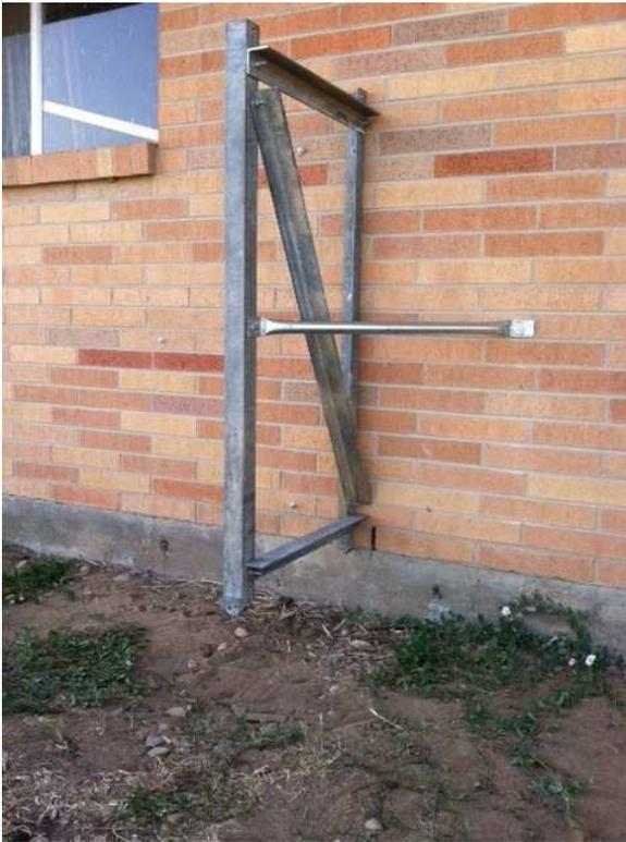
One limitation with this type of mount is that it doesn't provide a continuous attaching surface for the panel. The plywood back plate is what is bolted to the angle iron mount,
